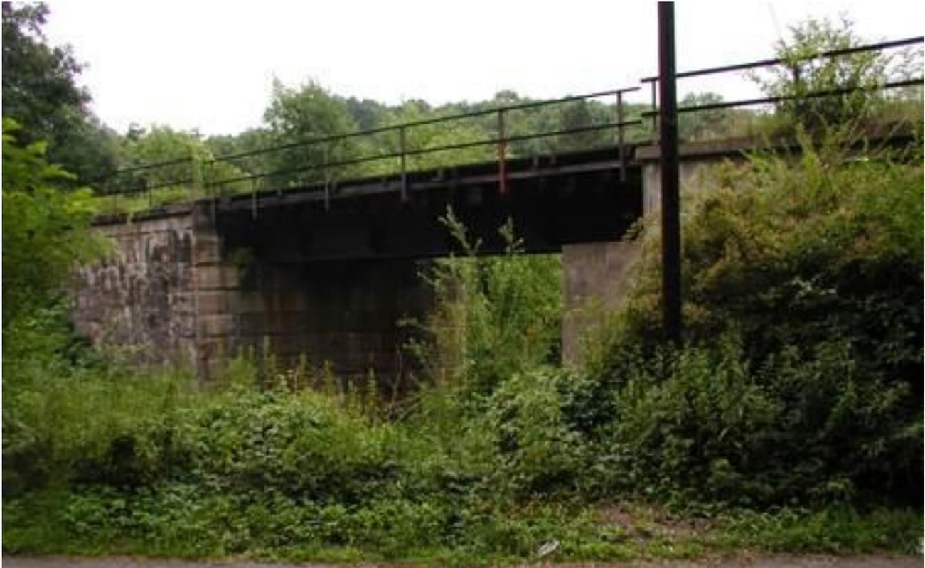
*We can find the original bridges these types in the places of crossing railway and road or small watercourse. The supporting parts of the bridge form typically 4 main beams which are connected by crossbeams with the supplemented runboard. The length of the bridge is about 5-10m. The bridge is sit at the abutment piers from stone blocks. The original grey painting is often overlayed by brown mixture of oil, rust, phenol and dust.*
